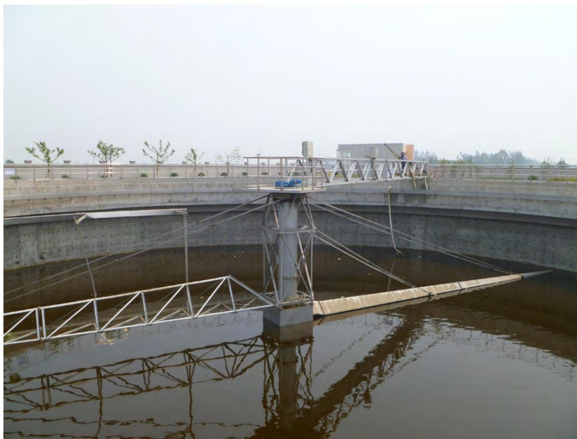
Central Driving perfectly solved the problems of clarifier edges leveling as well as driven trolley skidding in winter conditions.
