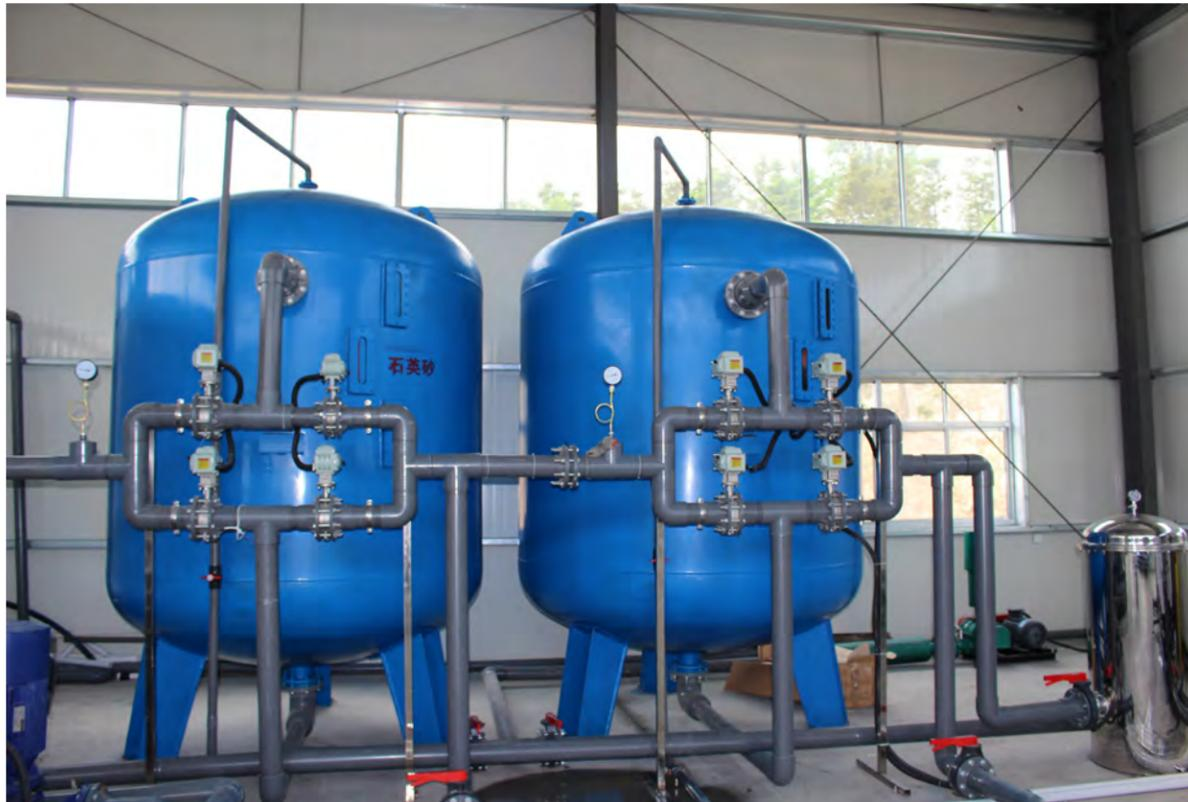
Raw water enters filter and is channeled to the filter top, and falls on a bed of filtration medium. Water get filtered from up to down under pressure while traveling across the filter bed.
